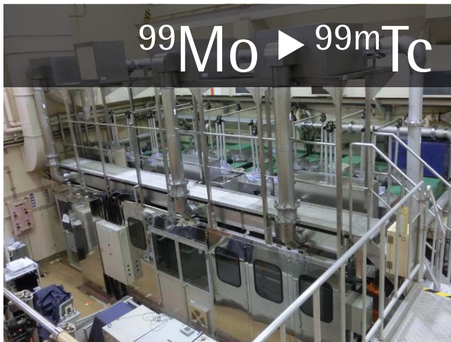
Clean booths installed at the JMTR hot lab
